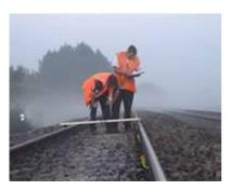
The image to the right shows engineers taking CANT readings whilst standing in the 4-foot during a T12 possession in the traditional fashion. In this scenario the engineers would be working in a green zone with all the extra manpower that this system requires.
