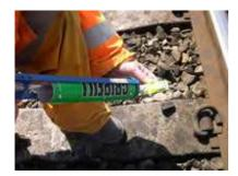
**Step One** — The base plate is affixed to the rail using approved adhesive and positioned on the wedge where necessary.
