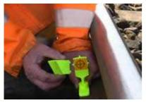
**Step Three** — The hood is positioned around the target to shield the target prism and protect it from fouling.
